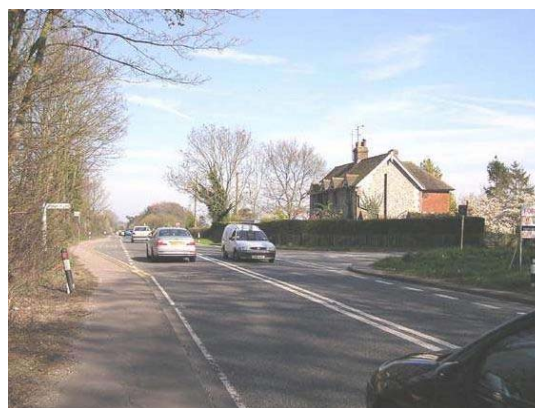
The existing A27 at Wilmington (image courtesy of the Highways Agency)
